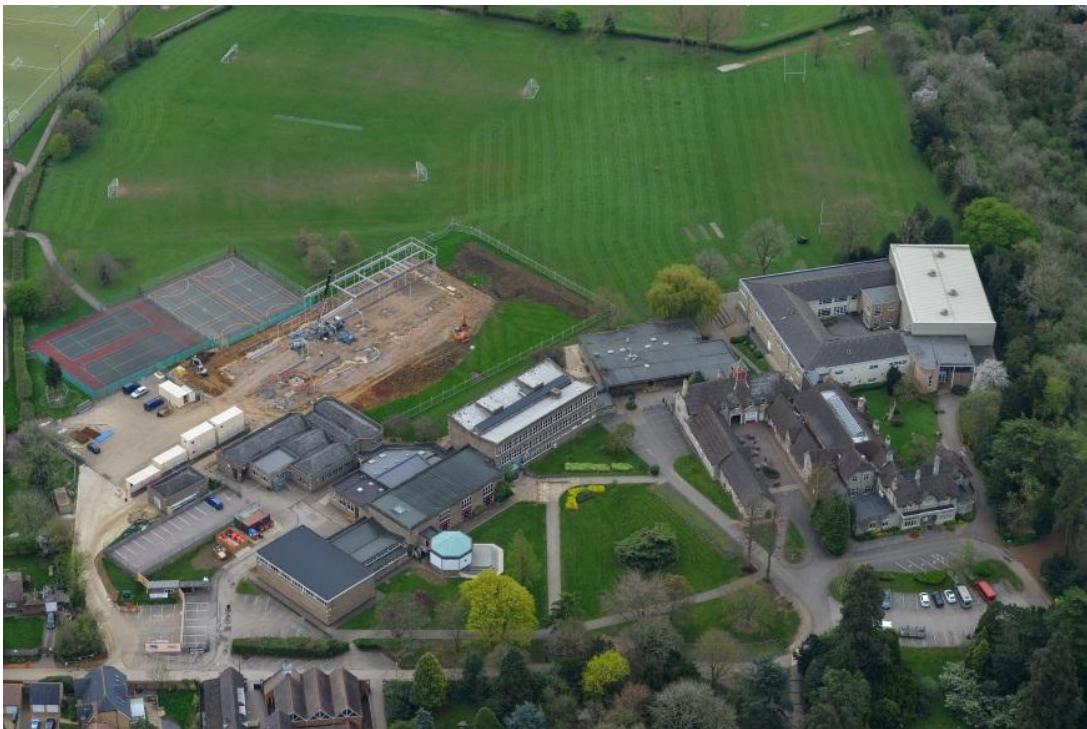
Royal Latin School, April 2014: construction of the Discovery Centre is under way
