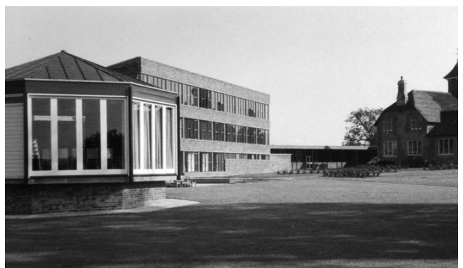
The new school building ('Main Block') on the Brookfield Estate in 1963
