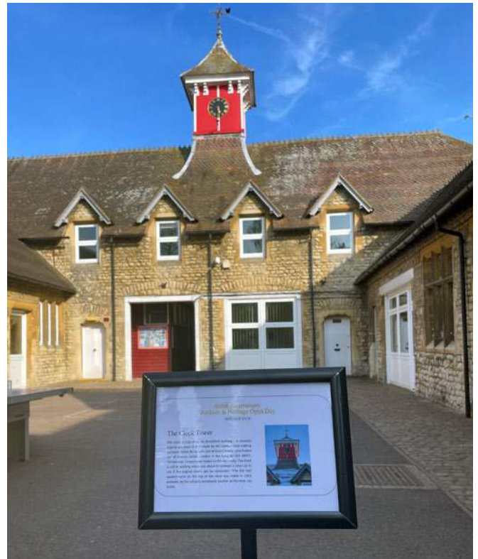
New details shared about the Brookfield Clocktower, restored this year
