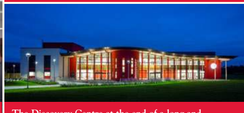
The Discovery Centre at the end of a long and memorable day (Photo: GSS Architecture/Fotohaus)
